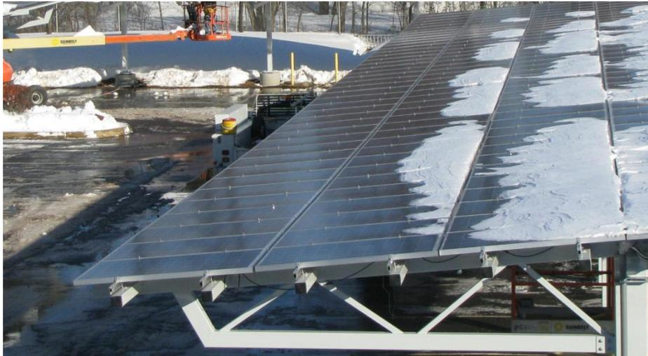
**5 degree slope, (standard) 8'-6" clearance structures 1 day after 22" snowfall**
